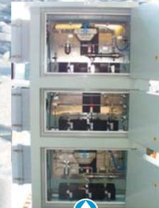
The superb thermal insulation properties of layered composite GRP makes it easy to design 'hot boxes' - to maintain elevated temperatures and prevent condensation or crystallization. INTERTEC can deliver optimized solutions with the right insulation, best form of heat transfer, equipment layout and control algorithm to ensure accurate, reliable performance.
