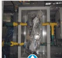
Highly insulated and heated enclosures allow explosion-proof equipment, rated for temperatures from  $-20$  to  $+40^{\circ}\text{C}$ , to be used in extremely cold environments - such as this design for a Siberian plant where the ambient temperature was below  $-50^{\circ}\text{C}$ .
