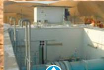
Advanced insulation is a key aspect of these shelters for the instrumentation/SCADA stations on a Middle East water pipeline, allowing totally passive cooling to limit the extremes of day and night temperatures.
