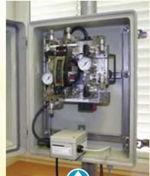
↑ INTERTEC produces several application-specific heaters such as this conduction heater for SP76 instrumentation substrates (mounted behind substrate).
