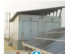
One of the largest passively-cooled shelters ever constructed - with a volume of 142 m<sup>3</sup> - for a Middle East pipeline project; 4 mm thick GRP sheets enclose 77 mm of insulating foam. The all-passive cooling shaves up to 20°C off peak daytime temperatures.
