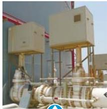
Special composite construction principles and insulation allow INTERTEC cabinets to keep critical equipment below 60°C for periods up to 120 minutes - to protect equipment such as emergency shut down valves.
